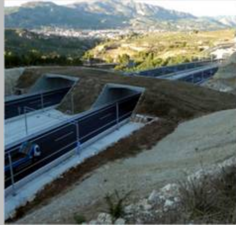
Photo 2 - Overpass details (© J. Juste)
